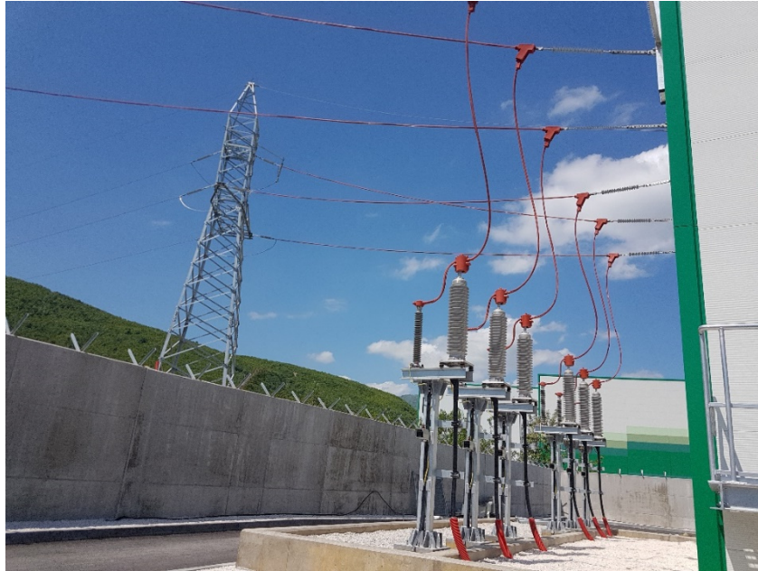
Fig.3 Overhead Line conductor cover
