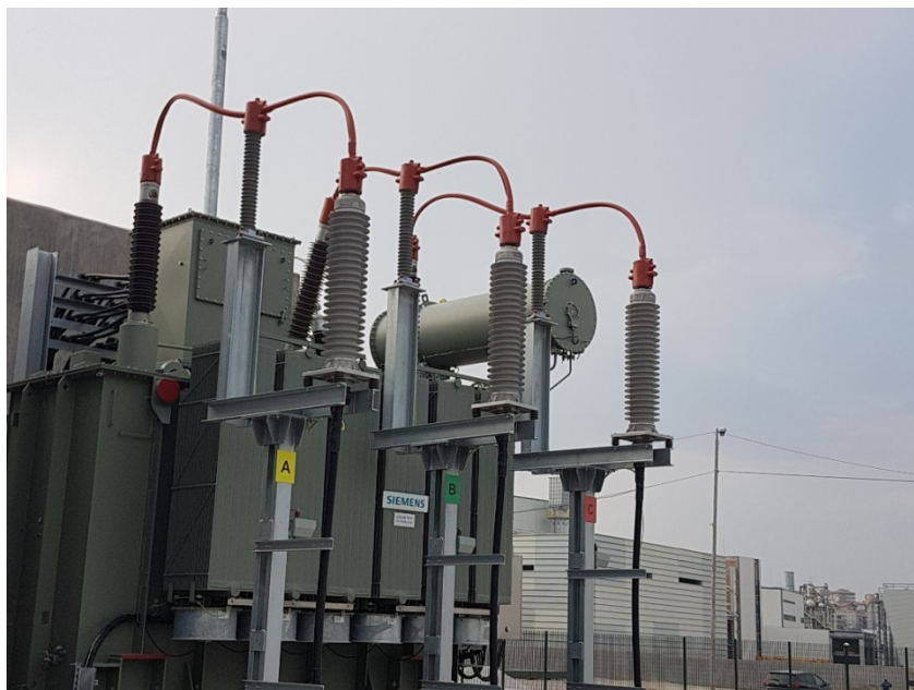
Fig. 4 Silicone cover of transformer 110 kV busbars
