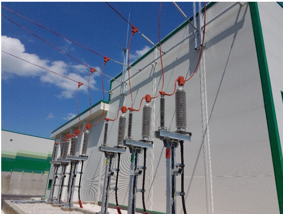
Fig. 2 Open plan 110 kV system
